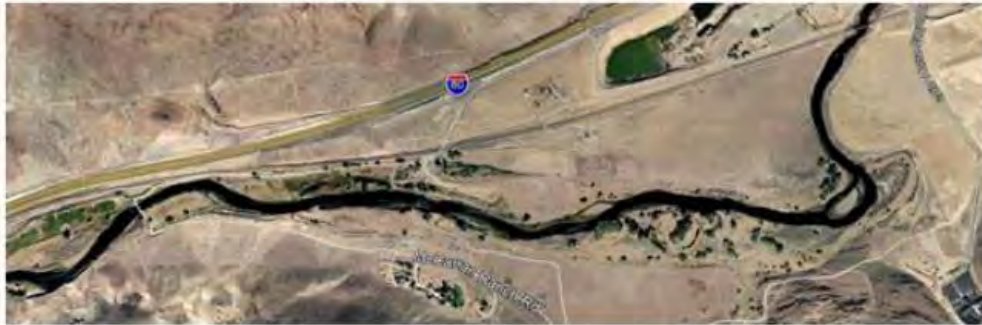
a. Pre-Construction – 16 September 2004
