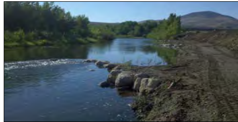
J-Hook Vane series following construction and willow planting Truckee River near Pyramid Lake
