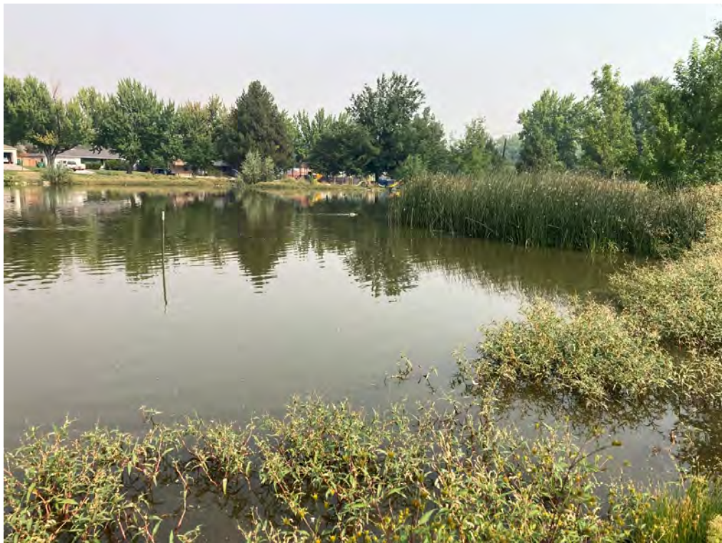
Lake Park, looking north at only section of reeds/cattails. Pole in water indicates return flow intake pipe.
