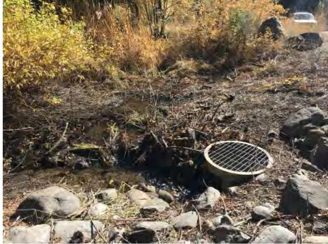
Standpipe blocks fish passage upstream from Incline Way
