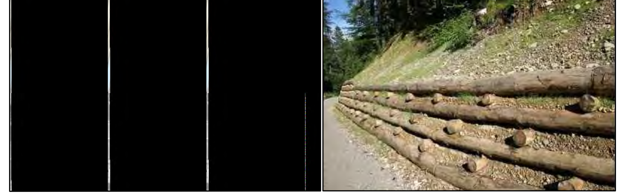
CRIB WALL BANK STABILIZATION/TRAIL ACCESS
