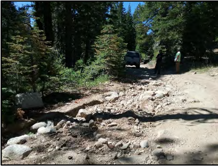
Photos (above) of steep dirt roadways in upper watershed without proper drainage contributing excess sedimentation to nearby waterbodies.
