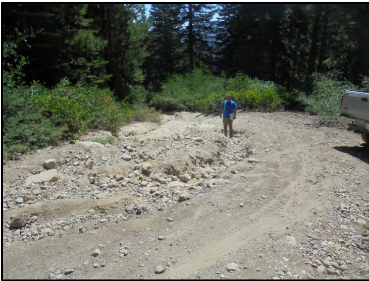
Heavy erosion causing rills and gullies along untreated roadway.
