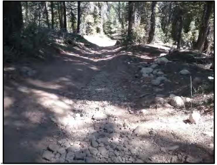
Photos (above) of steep dirt roadways in upper watershed without proper drainage contributing excess sedimentation to nearby waterbodies.
