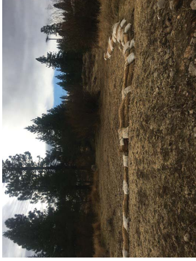
Figures 7 and 8: Site 5 on the floodplain of the Truckee River, before (Fig 7) and after (Fig 8) phase 1 construction. The project removed a concrete lined ditch (Fig 7), restoring the floodplain processes. These improvements will disperse and slow surface water. The majority of water quality improvements will have been made upstream of this site.
